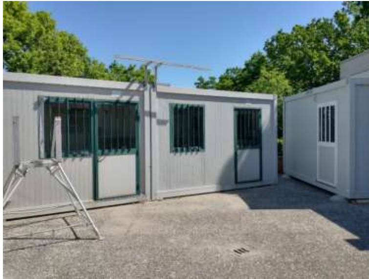
Figure 1. Monitoring station in Rende
